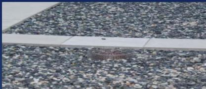
By slowly releasing stormwater to the sewer system, these controls increase the system's capacity, thus allowing WPCPs time to process and treat combined sewage and stormwater flows.
