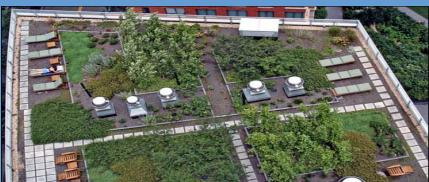
These vegetated source control techniques work through the infiltration of water to the soil and the transpiration of water by plants. They have the potential to withhold significant amounts of water from the sewer system and filter out or eliminate pollutants – acting as a network of distributed pre-treatment plants.
