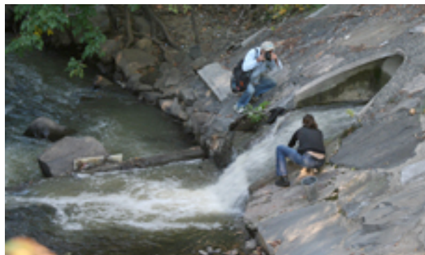
4.4 million gallons of sewage flowing into the Saw Mill River Photo courtesy of Bard Porchaska
