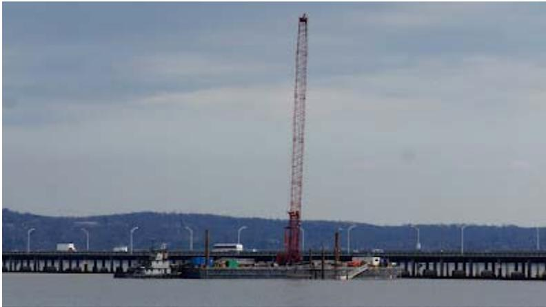
This equipment is driving test piles for the "Pile Installation Demonstration Project" (PIDP), seen in the image below.
