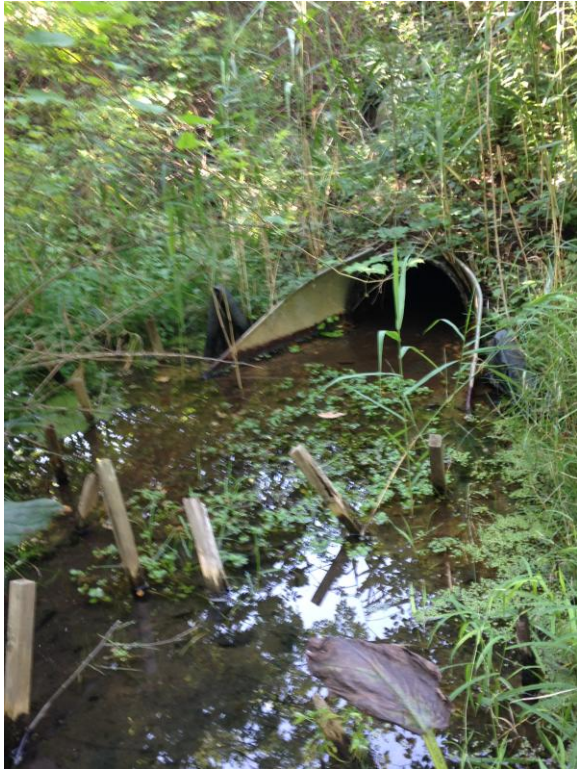
Westerly Outfall /c watercress
